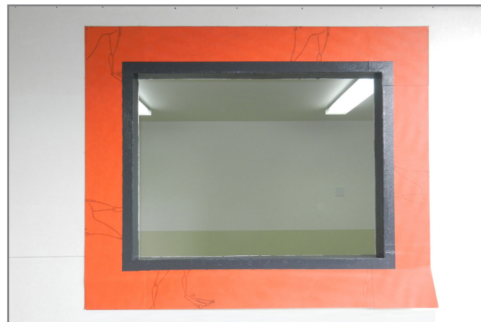
Completed application of VaproLiqui-Flash installed around all surfaces of rough opening.
