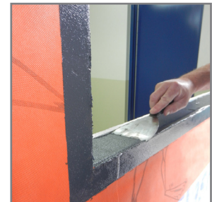
14. Allow VaproLiqui-Flash to set up until dry to the touch, then inspect for voids and apply additional VaproLiqui-Flash as needed to achieve complete coverage.
