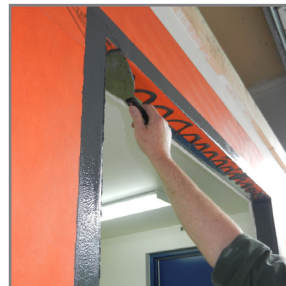
13. Immediately spread until all surfaces are completely covered and substrate below is no longer visible (approximately 12 to 15 wet mils).
