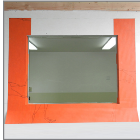
8. Install head flashing only after both left & right jamb pieces are fully adhered.
