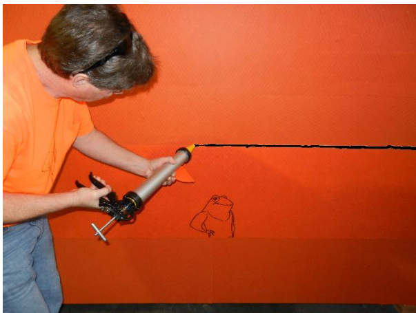
Apply VAPROBOND at a minimum 3/8" bond line to the reverse lapped membrane.
