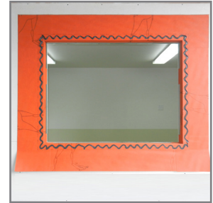
10. Using the sausage gun, apply VaproLiqui-Flash in a zigzag pattern on the wall face surrounding the rough opening.
