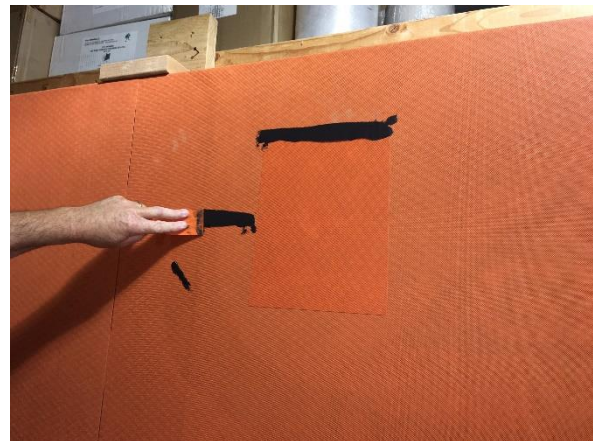
Apply VAPROBOND to the abrasion and reverse lap of the patch to ensure a water and air tight seal. Use a DRY joint knife, trowel, or spatula to tool sealant.
