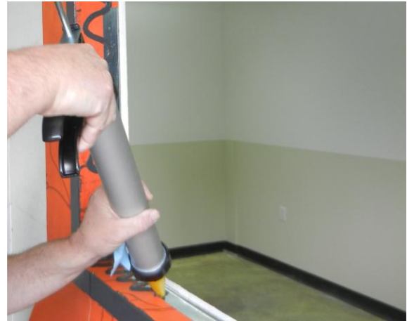
Apply using a professional caulking gun.
