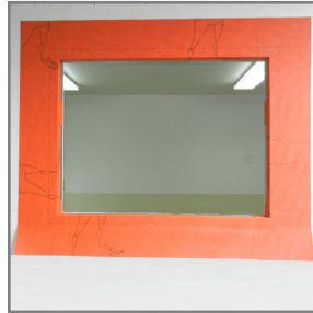
9. Repeat steps 4 and 5 for the head flashing.
