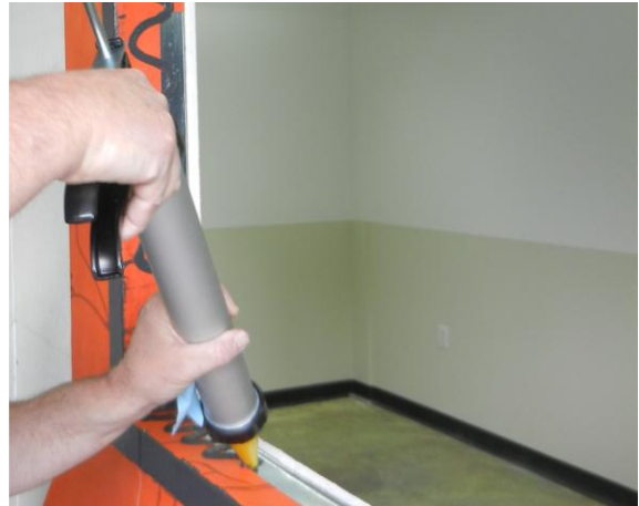
Apply using a profesional caulking gun.
