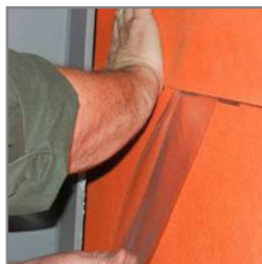
10. Use the opposite hand to smooth the two layers together as the release film is removed.
