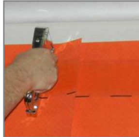
2. Install with SS staples in the top 2" above the Integral Tape. Avoid stapling in the tape area.
