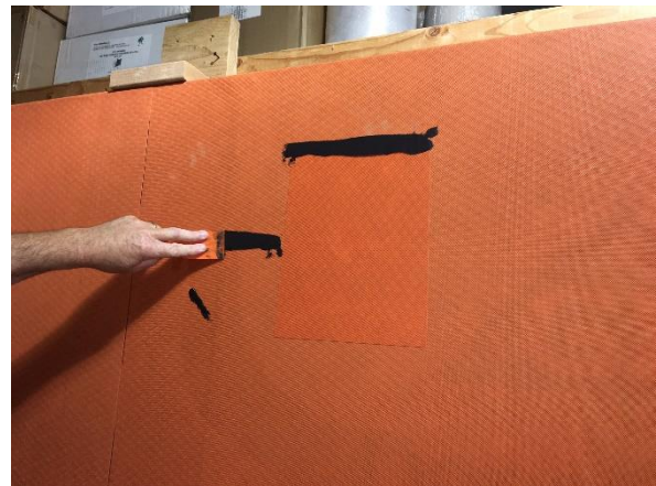
Apply VAPROBOND to the abrasion and reverse lap of the patch to ensure a water and air tight seal. Use a DRY joint knife, trowel, or spatula to tool sealant.
