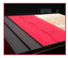
Immediately install metal roofing material onto each vertical run of SlopeShield.
