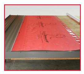
Metal roofing material should be installed immediately to each vertical run of SlopeShield.
